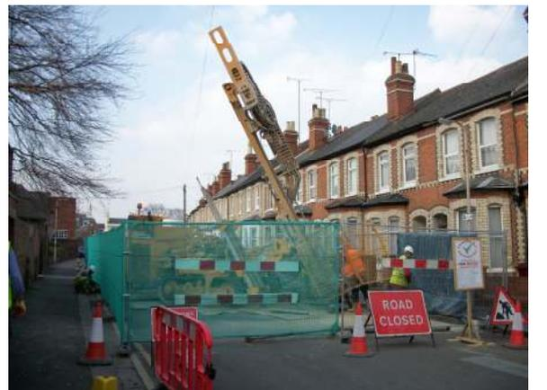
During the investigation and stabilisation work continuous monitoring of properties was carried out using laser levelling, precise levelling, EDM surveys, crack monitoring 'tell tales' and physical condition surveys.
