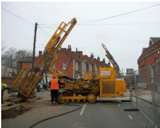
We used inclined drilling techniques for much of the drilling under the properties so we could carry out the work from roads, gardens and courtyards around the buildings, rather than carry out any of the work from inside properties which would have been immensely disruptive, and we used several rig types to ensure we could cope with the varied access restrictions.
