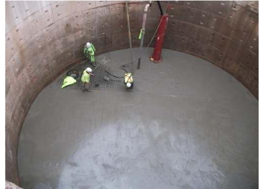
The shaft base plug was poured with the assistance of divers to place the non-wash out concrete mix.
