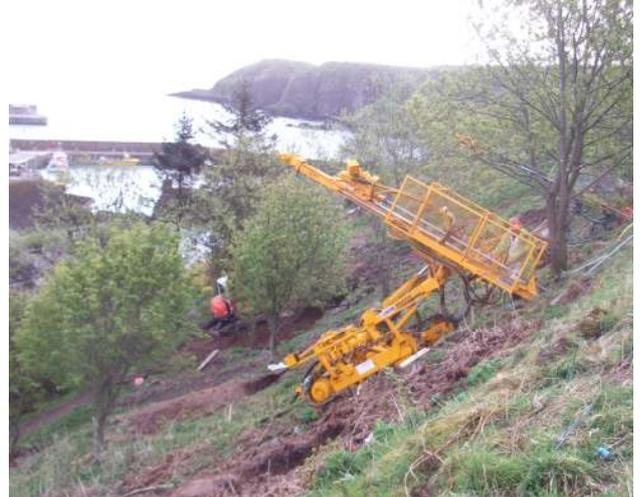
The length and steepness of the slope, the restricted access to the base of the slope together with the large number and length of soil nails meant that conventional soil nailing equipment including excavator mounted feed beams or rope access equipment was not suitable for this location and we established an innovative system of tracked, air powered rotary percussive drilling rigs secured and hauled by winches which were set up on the closed Bervie Braes road.
