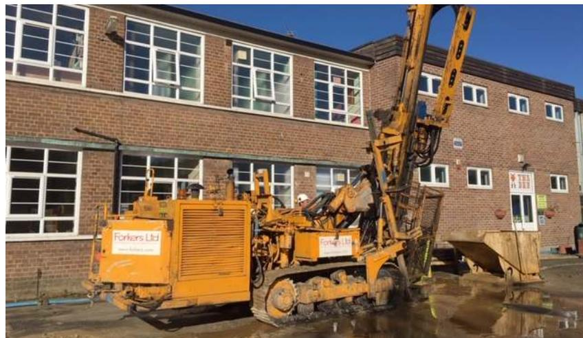
**Treatment works Phase 3.** The treatment phase of the project used 2 drilling & grouting methods;
