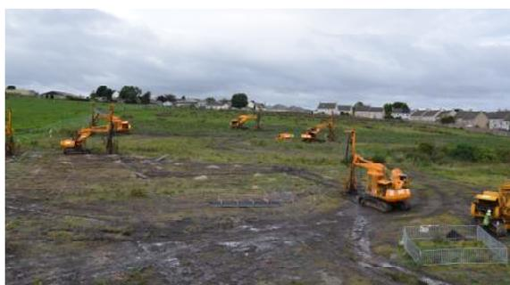
During the works up to 10 drilling rigs were resourced to site together with 2 grout mixing plants and at peak production over 40 operatives were on the site. All drilling and grouting plant and equipment was resourced from our specialist in-house plant fleet.
