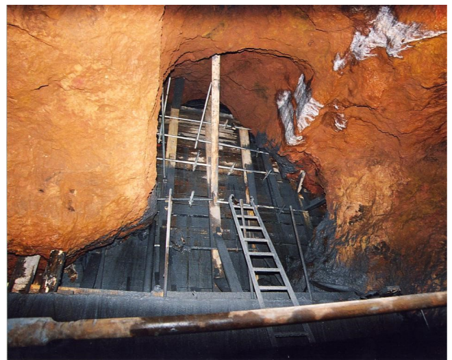
Shuttered barrier and grout infill area
