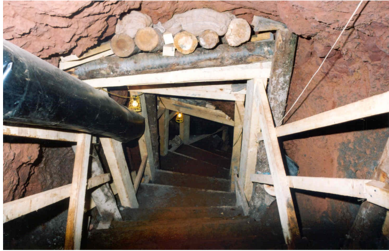
Access adit to Rough Winds Mine
