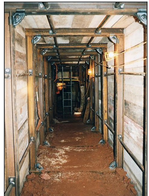
Permanent roadway through infilled mine
