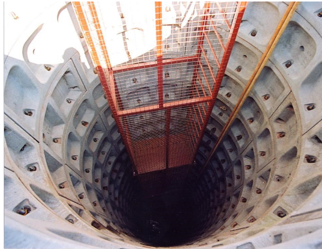
Access shaft to Brooklyn Mine
