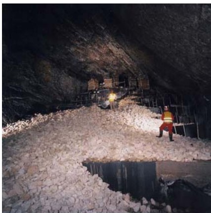
Northern Gallery showing supported working platform, barrier steps, and infilled limestone.
