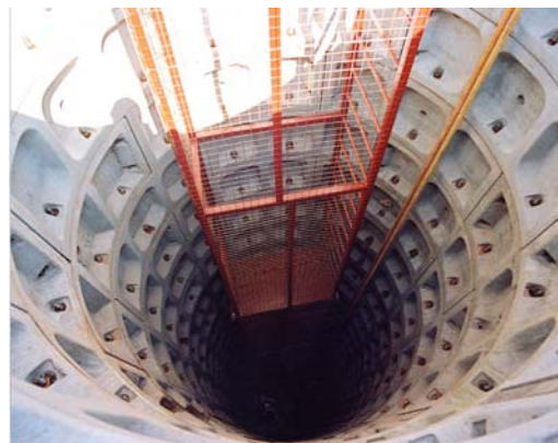
Access shaft to Brooklyn Mine
