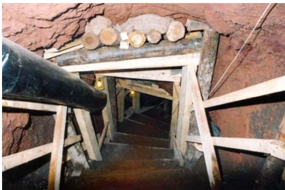
Access adit to Rough Winds Mine
