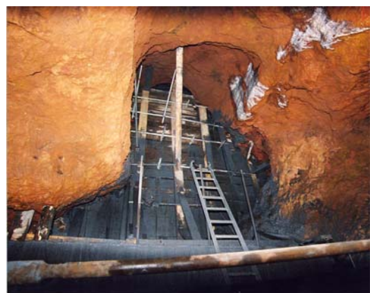
Shuttered barrier and grout infill area
