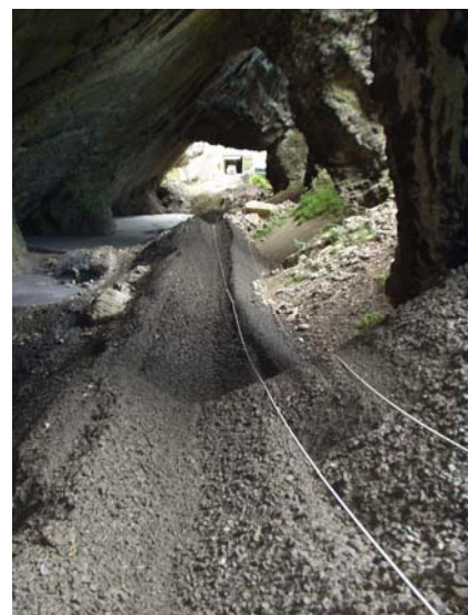
View through gallery at start of stone infilling
