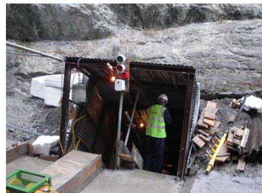
View of tunnel portal
