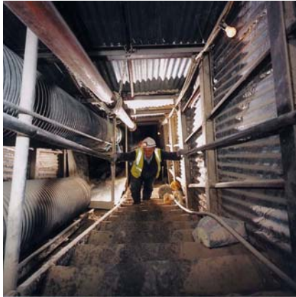
View down completed tunnel
