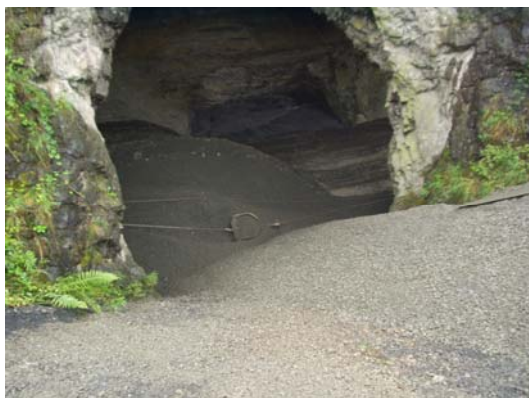
'Slusher' distributing infill stone
