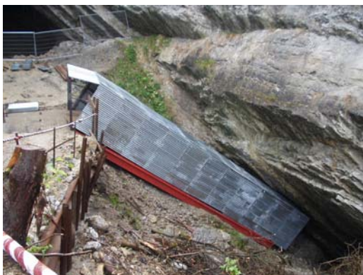
Tunnel portal section prior to filling over
