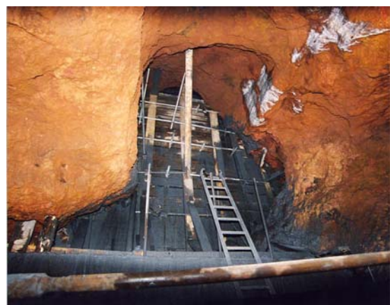
Shuttered barrier and grout infill area
