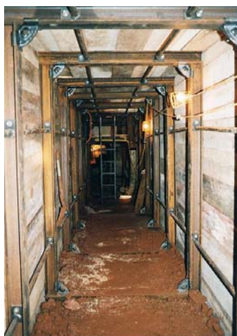
Permanent roadway through infilled mine
